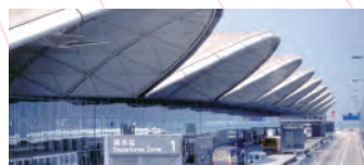
Hong Kong International Airport
